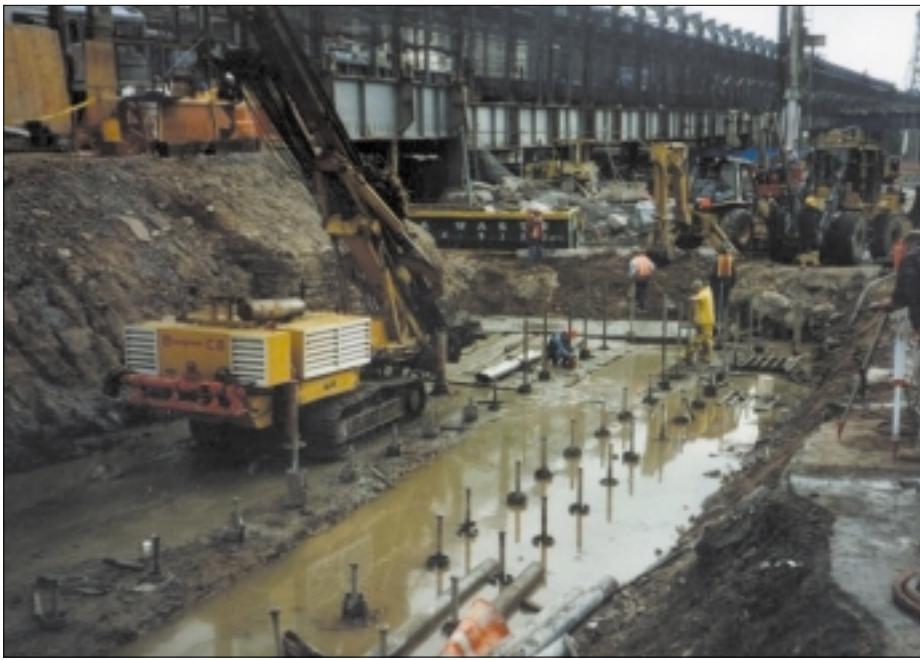
Work-site congestion and overcrowding can significantly impede productivity.
